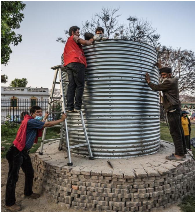
Oxfam staff and volunteers construct an 11,000 litre water tank at Tundikhel IDP camp. Oxfam is providing water to 15,000 people here. Photo: Pablo Tosco / Oxfam
